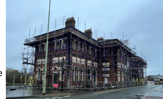
2022 – March, scaffolding erected due to deterioration of corbels
